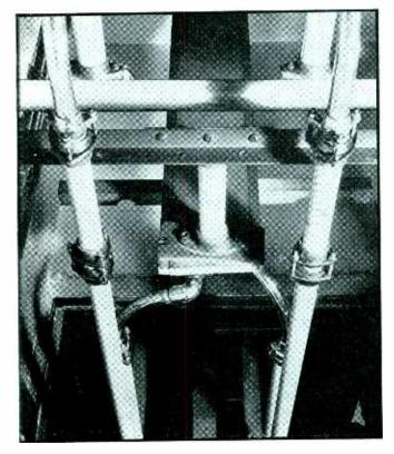
Fig. 3—Method of making bends with copper tubing and bronze fittings
