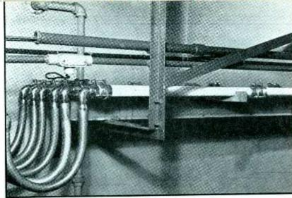
Fig. 4—Pipe ends with lead expansion loops connecting them to the pumps
