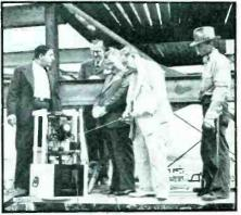
A portable transmitter, with an induction heating coil attached in place of the antenna, was used to heat the last rivet in the steel work of the RCA Exhibit Building at the New York World's Fair Grounds. The rivet, suspended in the induction coil, became white hot in less than a minute
