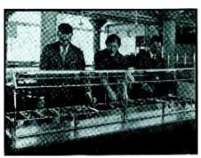
Ultra - violet - producing Sterilamps have been installed in the cafeteria of the Westinghouse Lamp Division to irradiate tableware. The ultra violet wavelengths used lie in the so-called "bactericidal" region of the spectrum
