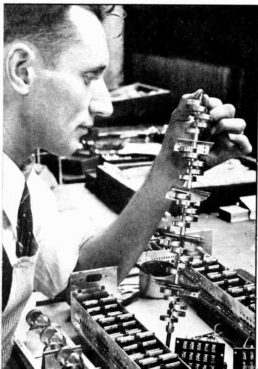
Cam mechanism used in Super-Pro switch mounted eccentrically actuates Bakelite sections with silver plated knives. Switch is over 12 inches long; weighs nearly 3 pounds
