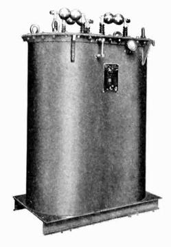
Left—AmerTran inverse feed-back modulation transformer for service in a 50 Kw. high-level broadcast transmitter.
