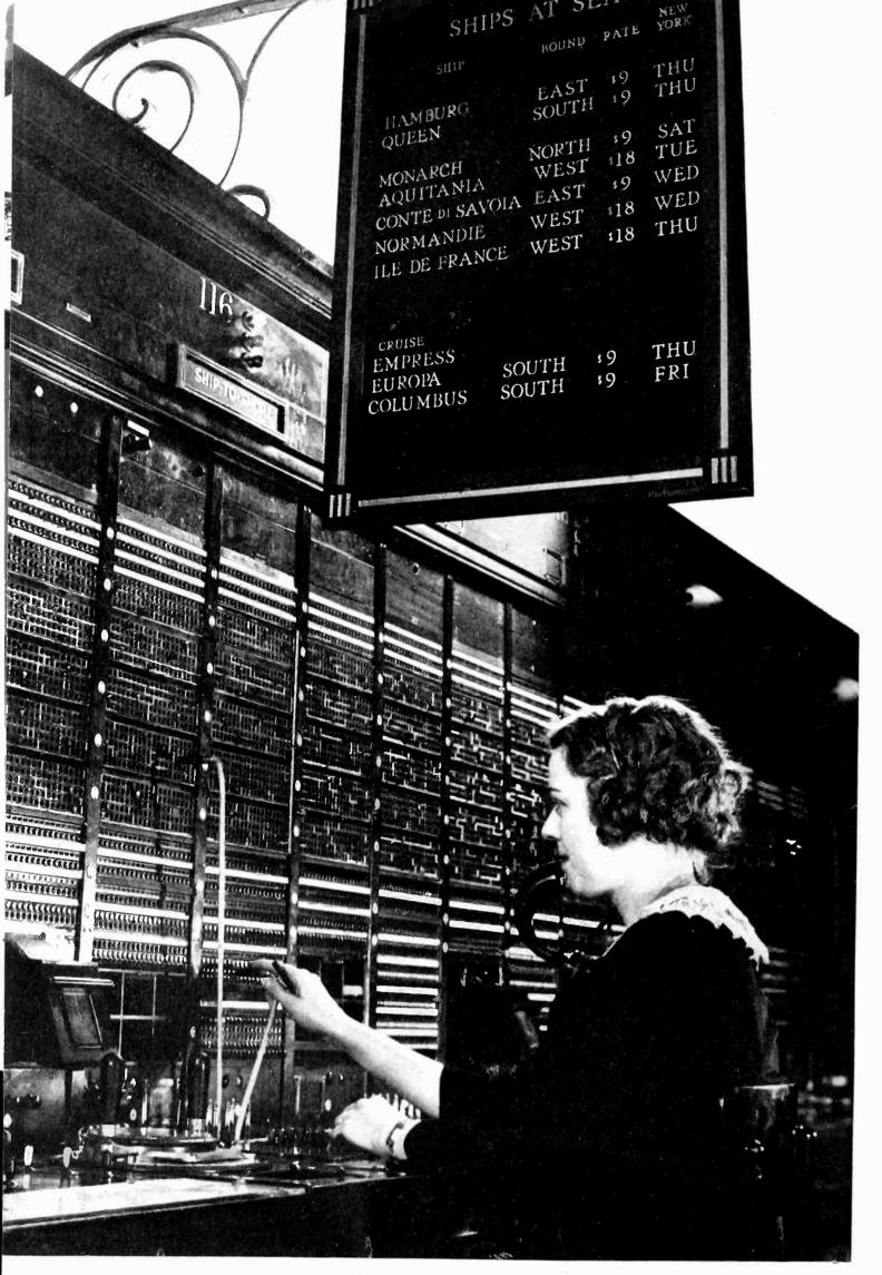
Toll operator putting through ship-to-shore call at 32 Walker St., New York City, from which position connection can be made with 34,000,000 telephones in 68 countries
