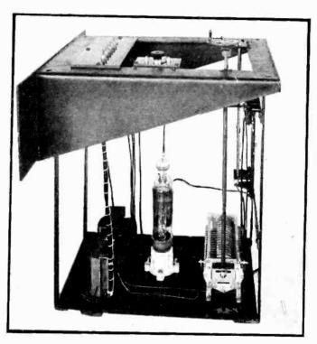
Fig. 5—Simplicity is the keynote of the interior of the voltage regulator
