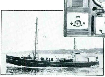
Radio aids the fishing fleet. The Rio Duoro, out of Gloucester, finds the fishing banks by following compass signals. The installation (inset) includes, at the left, a marine all-band radio receiver for news and entertainment
