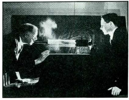
G. W. Penney (left) and L. W. Chubb of the Westinghouse Laboratories examining a high-voltage dust remover. The dust becomes ionized in the presence of a high electric field, and is attracted to the charged plates. The device is expected to be of value in the treatment of hay fever
