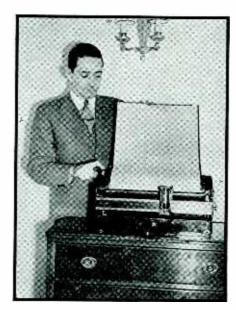
Sound recorded photoelectrically in parallel lines on photographic film is transferred to metal and printed on ordinary paper, from which it can be reproduced by a phototube pick-up, shown above
