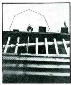
Berlin's "pancake" television radiator, 453 feet high, which sends video images on 6.7 meters. The "edges" of the pancake are horizontal dipole elements which concentrate the energy in the horizontal plane
