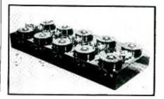
Nearly 1500 different types of noise are claimed for this German film-and-phototube device which contains five complete reproducing units. Used separately or in combination, the noise outputs are amplified and used for broadcast and motion picture applications
