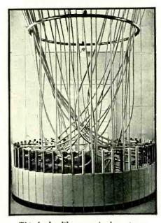
This basket-like maze is the antenna termination system of the German directional receiving station at Beelitz. The circular base permits switching on any of the 54 lead-ins, each of which can feed three receivers
