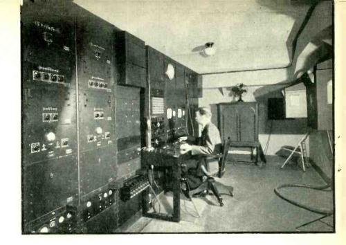
The film-projection room is fitted with monitoring apparatus for two video and audio channels, one for each projector, so that continuous film programs can be handled.
