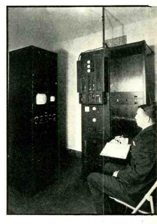
The radio relay transmitter at the RCA Building which transmits the video signal on 177 Mc. to the main transmitter in the Empire State Building
