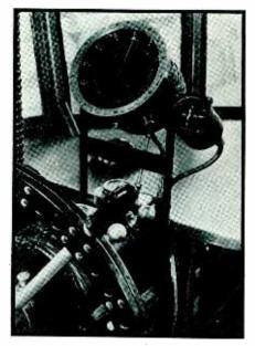
small indicator is for use with the blind-landing radio beam, for guiding the new zeppelin through fog
