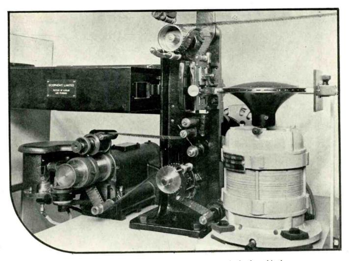
Close up view of the high speed scanner and motor, projector head and sound head showing a film threaded up ready for operation
