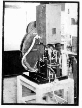
Television transmitter and receiver built by T. Sone of Tokyo. The disc method is used
