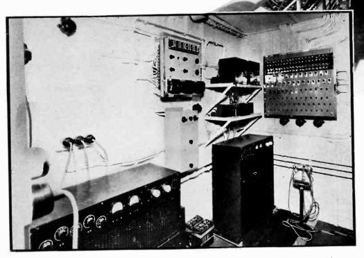
Views of the control room from which records are played. Power equipment, turn tables, amplifiers, loud speakers were supplied by Philips.
