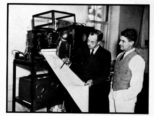
Dr. Harlan Stetson, and Thomas S. McCaleb of Harvard with an automatic signal-strength recorder. The record indicates that the moon as well as the sun causes changes in ionization of the upper atmosphere
