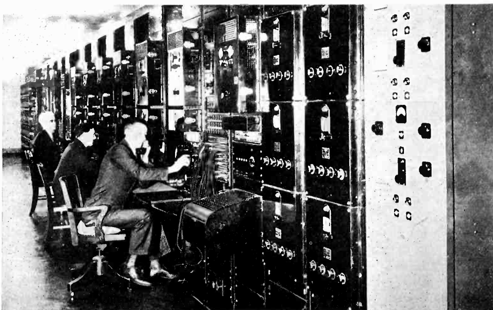
View of the radio program distribution equipment of the Waldorf-Astoria Hotel in New York. Among the six program choices provided for guests are several European shortwave programs
