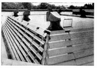
Adjustable louvers on skylights, which are automatically opened or closed to provide sufficient illumination but no glare in the sorting room below
