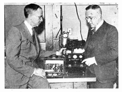
A photocell, held by A. H. Taylor activated by UV passes current into a condenser where it is stored to be released in spurts to be counted. This electronic device was developed by Mr. Taylor and Dr. Matthew Luckiesh of Nela Park
