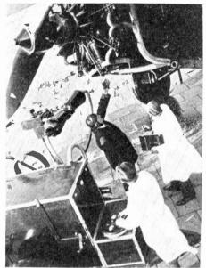
At the Fuhlsbuttel aerdrome near Hamburg, Germany, a portable X-ray outfit can be wheeled out onto the field and used to inspect propellers, engine parts, and gear, detecting flaws invisible to the eye
