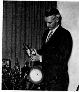
Utilizing a sensitive millivoltmeter Mr. R. C. Hitchcock measures the voltages produced by various fruits and liquids
