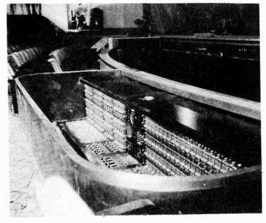
The lighting-control box in the pit of the large theater, with its 2000 control knobs
