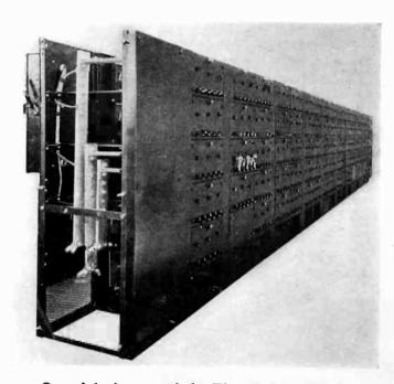
One of the long panels for Thyratron control circuits in Music Hall. Reactors are directly behind tubes
