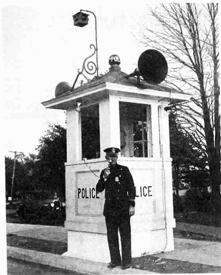
Short-wave police systems increased rapidly in 1932. Now photocells detect speeders. And here's the latest, a microphone feeding loudspeakers a quarter mile away, so the policeman can instruct drivers as far as he can see them
