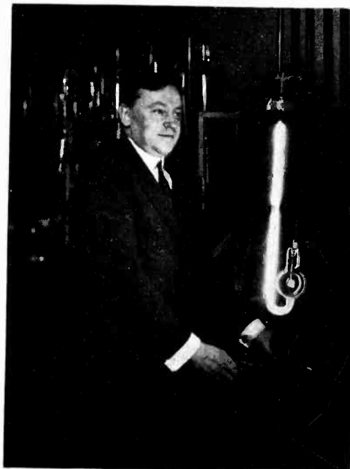
Dr. Harvey C. Rentschler, director of research, Westinghouse Lamp Company, experimenting with the new highly efficient hot-cathode positive-column zinc arc, produced by passing current through a mixture of argon gas and zinc vapor
