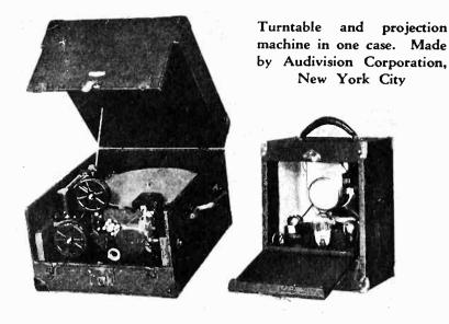
Present home sound movie equipment is designed for the professional 16 inch  $33\frac{1}{3}$  r.p.m. disc, while in some cases, the turntable can be used for commercial 78 r.p.m. records. The complete sound unit is designed to operate off 110-volt 60-cycle a.c. with no additional batteries required. Specifications for the projector lamp are similar, usually requiring one 20-volt 250-watt lamp. A special transformer is supplied to furnish this voltage from the 110-volt circuit.
