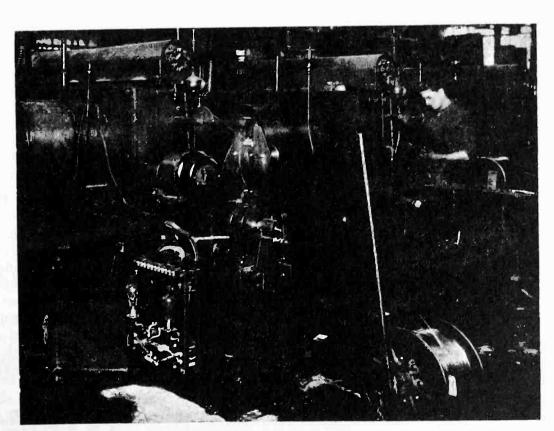
Electronic tubes keep uniform the tension on this wire as it is reeled onto spools in layers of constantly increasing diameter
