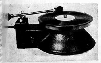
This turntable, manufactured by the Hollywood ilm Enterprises, is designed to connect to standrd 16 mm. silent projectors by means of a flexible shaft
