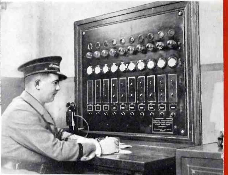
Above—Electric Eye—Traffic Control Room on the Ambassador Bridge at Detroit. System illustrated devised by Benjamin Cooper of New York.
