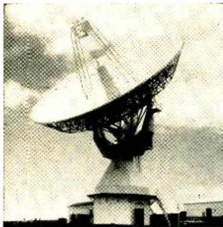
This 85-ft antenna at the earth station at Paumalu, Hawaii has served as gateway station to the mainland. The facility has been recently expanded with an additional 96-ft antenna for Pacific traffic.
