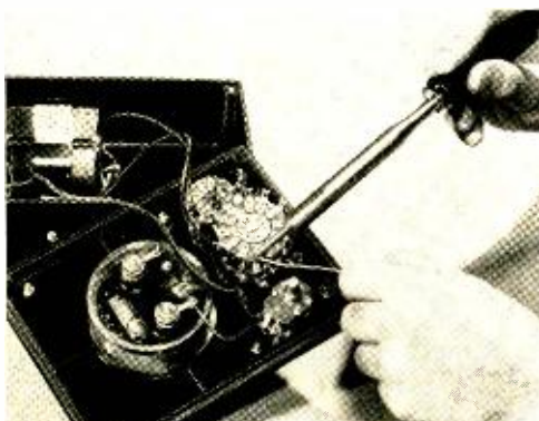
Construction of Multimeter.
