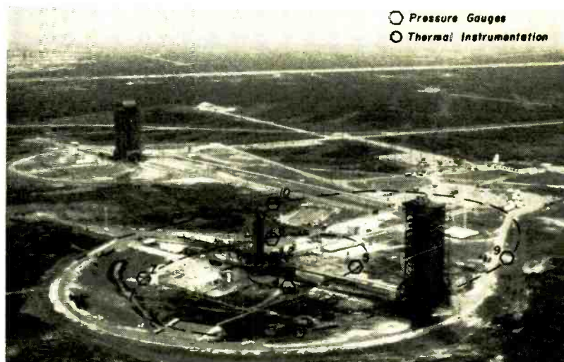
The over-all view of Launch Complex 36 at Cape Kennedy with the location of the pressure gauges and thermal sensors indicated.
