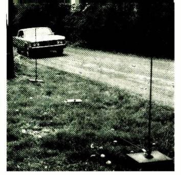
Fig. 3. An experimental **RRA** roadside transmitter system. Permanent installation would be on high, fixed supports.
