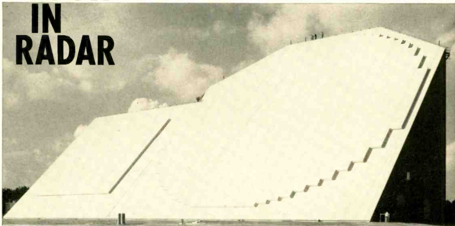
Fig. 1. The newest and largest of the phased-array radars. The array is 327 feet long, 145 feet high, and 145 feet wide.
