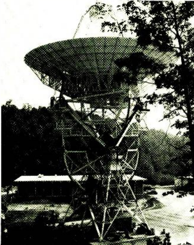
This 85-ft. antenna, located at the Rosman, N.C. tracking and data acquisition site, will be used with NASA's "second generation" vehicles such as the Nimbus weather satellite. A permanent staff of 75 people is needed to run this tracker site.
