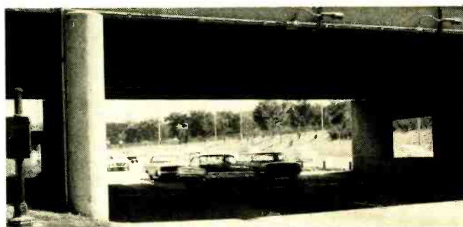
Overhead ultrasonic vehicle-presence detectors, part of Chicago's Congress St. Expressway traffic-surveillance system.
