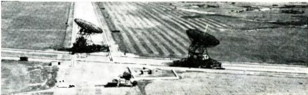
Both parabolic antennas of the Royal Radar Establishment telescope are on tracks.
