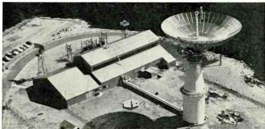
Lincoln Laboratory's Radar Observatory at Westford, Mass. Venus was "seen" with the maser-equipped dish at the right. Frequency used was about 300-500 mc.; pulse power was 265 kw.; dish size was 84 feet. Maser is at feed point of dish antenna.
