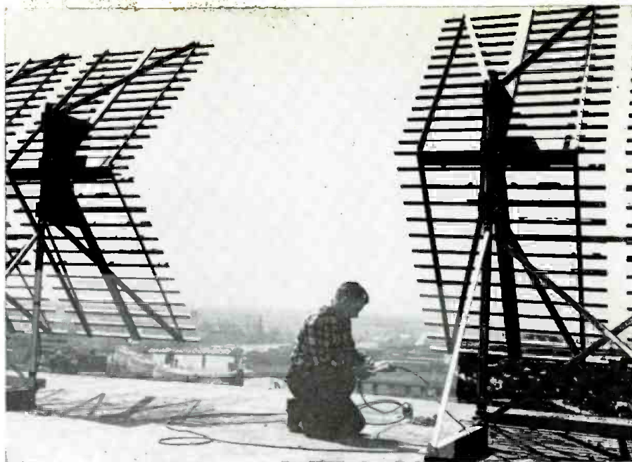
These reflectors face a similar pair located some 69 miles across the open sea.
