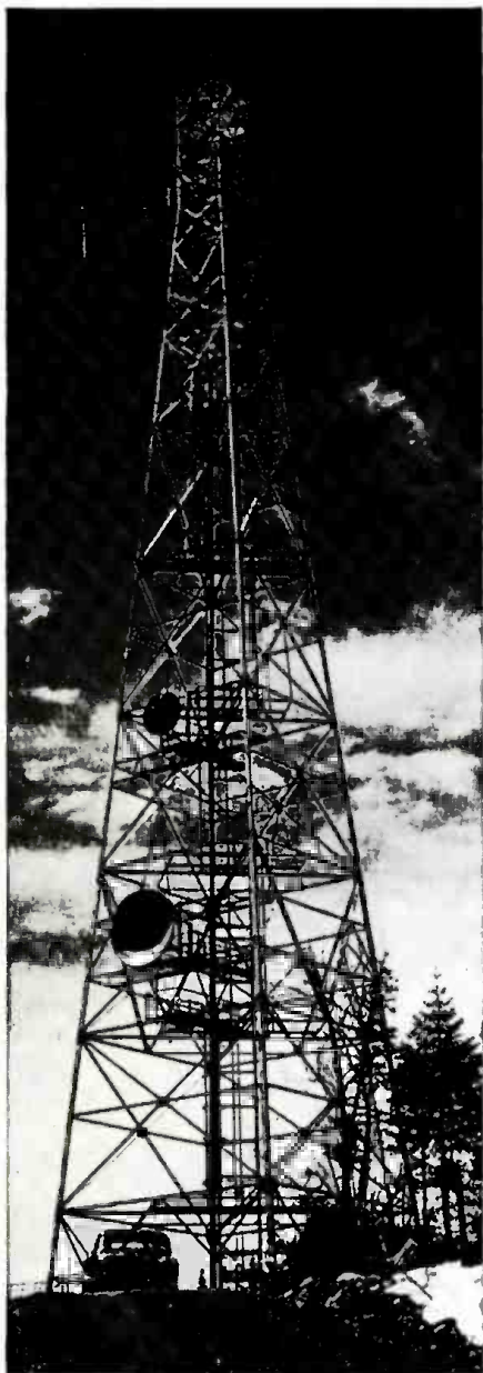
This hill-top installation at Deer Lake is typical of Newfoundland's repeater stations.
