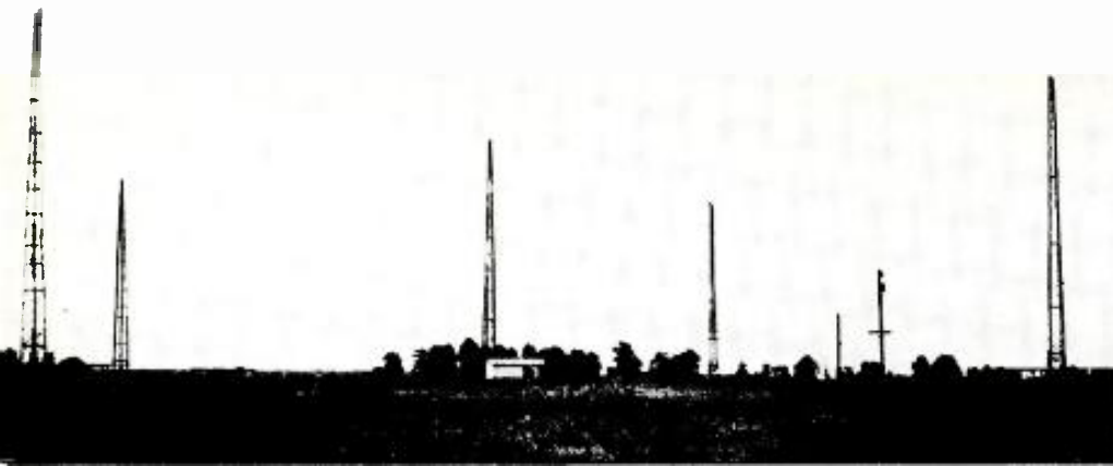
Four-course low-frequency radio-range station showing the five antenna towers.
