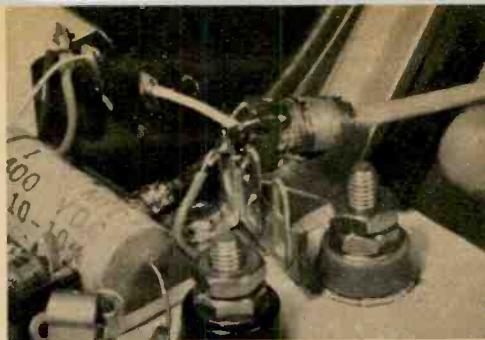
Fig. 4—To peak T1, supported by soldering its lugs to terminal strip, set up for FSM measurements and adjust the slug with alignment tool.
