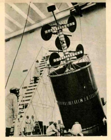
Tactical Satellite? ... The Air Force Space and Missile Systems Organization now has a new baby to play with. It's an experimental communications satellite-the largest and most powerful everbuilt by Hughes Aircraft. The monster is as tall as a two-story building and will be launched from Cape Kennedy into a synchronous orbit aboard a Titan-3 booster. This rotund fellow can handle 10,000 telephone channels and pop them into dish antennas only 1 ft. in diameter.
