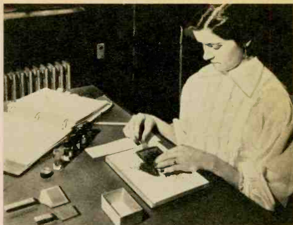
Tiny computer memory cores are counted with a paddle containing 400 holes. Worker scoops up cores, makes certain every hole is filled.
