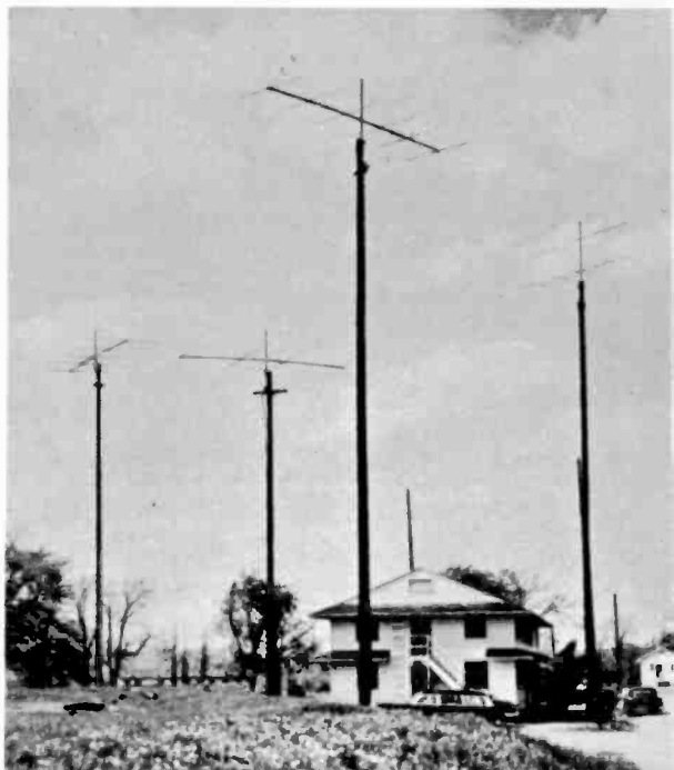
Antenna farm at Fort Monmouth, N. J., (K2USA) features several Telex beams for different bands. Shack has antenna patch panel. You can use simple dipole for 20 meters.
