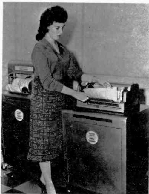
Western Union's coast-to-coast facsimile service is now available to all. Operator sets up letter on scanning unit while incoming fax copy arrives in basket of companion machine.
