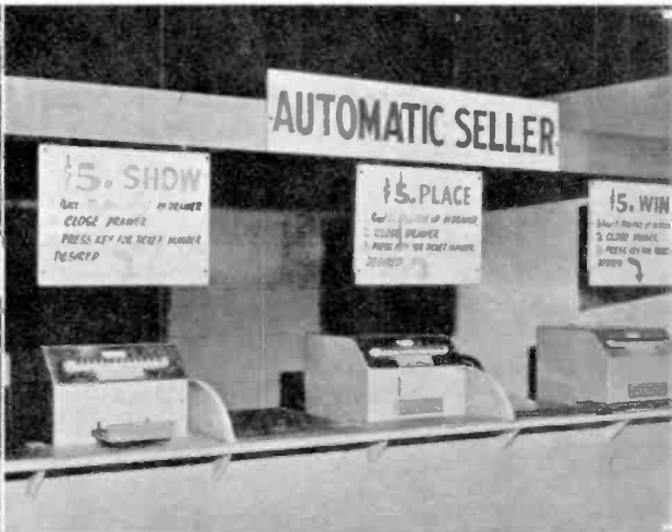
Amteller, now in use at Yonkers Raceway, is automatic ticket seller. Customer puts bill, face up, in money drawer, closes it and presses one of 12 buttons to indicate his choice. Photo-electric scanner certifies bill, issues pari-mutuel ticket.
