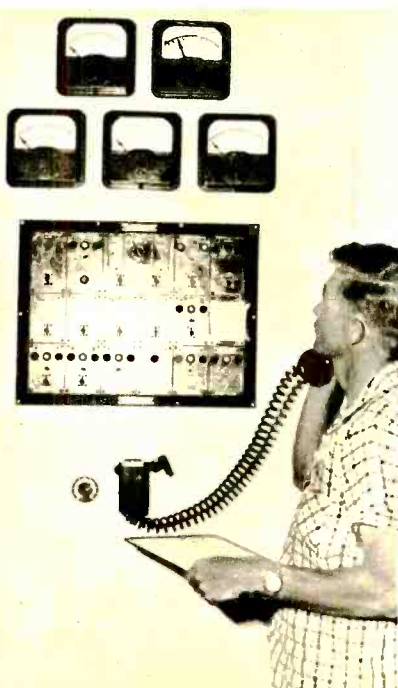
Small, simple control panel can govern huge water gates on the distant dam to meet irrigation schedules.
