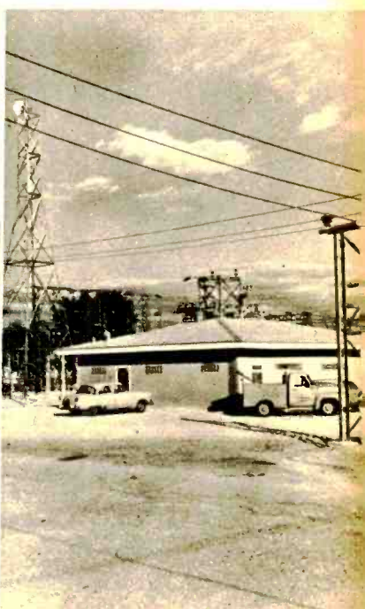
Mesa switching station is surrounded by power lines. Remote control equipment is housed in this low building.
