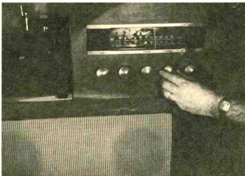
Switch inputs to isolate the trouble. Above, loud ringing occurred when using phonograph. The cabinet was sending vibrations back to pickup arm.
