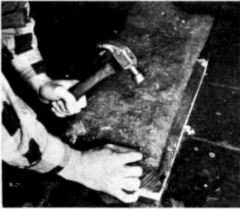
Tack Fibreglas insulation, old towels, etc., to the inside of the back and sides of the enclosure to absorb undesirable sound waves.
