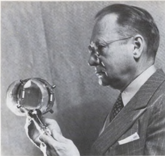
1929—The father of electronic television, Dr. Vladimir K. Zworykin, with his two basic inventions—the iconoscope camera tube (left) and the kinescope picture tube in an early receiver (right).
