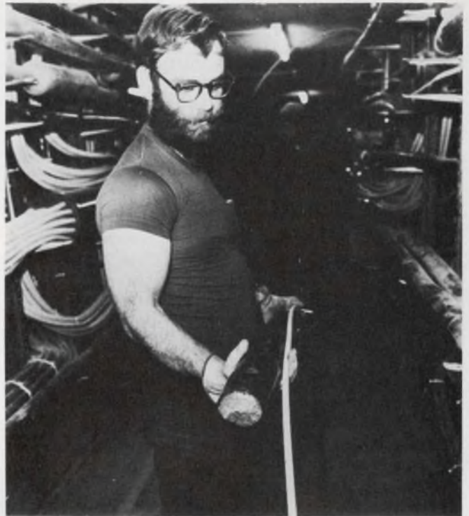
1977—An Illinois Bell lineman compares the new 1/2-in. optical cable installed for the Bell System's tests in Chicago with the large wire cable it replaces.
