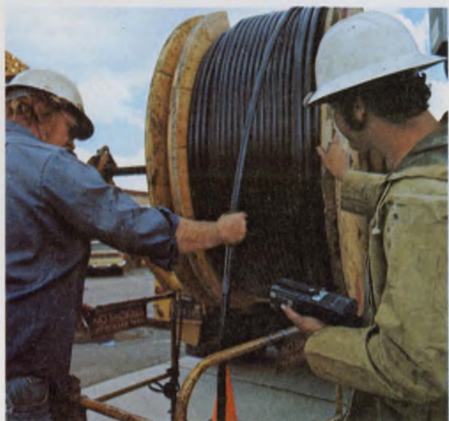
1977—Special fiber-optic cables developed to withstand the rigors of being yanked through telephone manholes and conduits have been put in General Telephone and Electronics' operating optical communications system in Long Beach, California.
