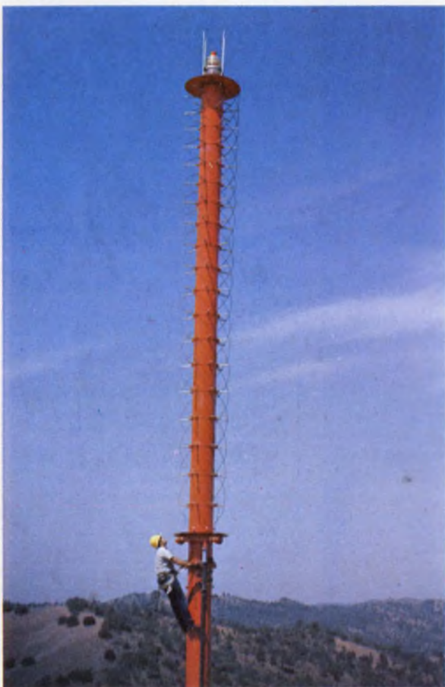
Circularly polarized TV transmitting antenna , located on Mt. Oso, west of Modesto, CA, has a CP power-gain ratio of 16 and is capable of 220 kW of input power. Built by Jampro, a subsidiary of Cetec Corp., Sacramento, CA, this is said to be the first CP antenna to be used for TV.
