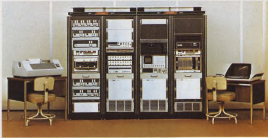
Writing and debugging of programs can be accomplished while PC boards are simultaneously tested on this Systron-Donner 3600 Computer Automated Test System. It uses a Basic operator interactive test language.
