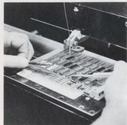
Impulse-bonding system developed by Bendix uses Teflon-coated, nickel wire for PC board interconnections.
