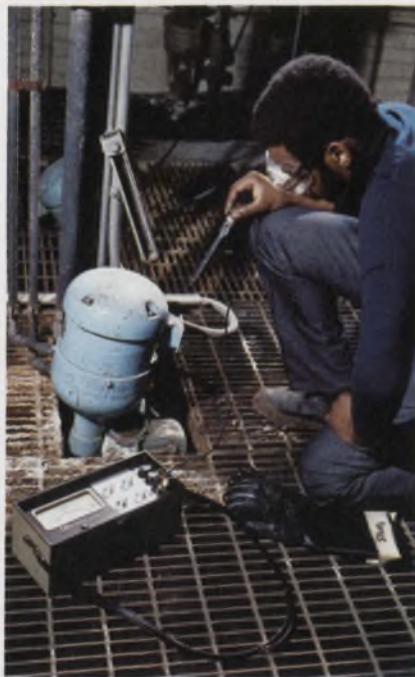
Measurement of waste-water pH with Leeds & Northrup tester gives a check for water-treatment operation.
