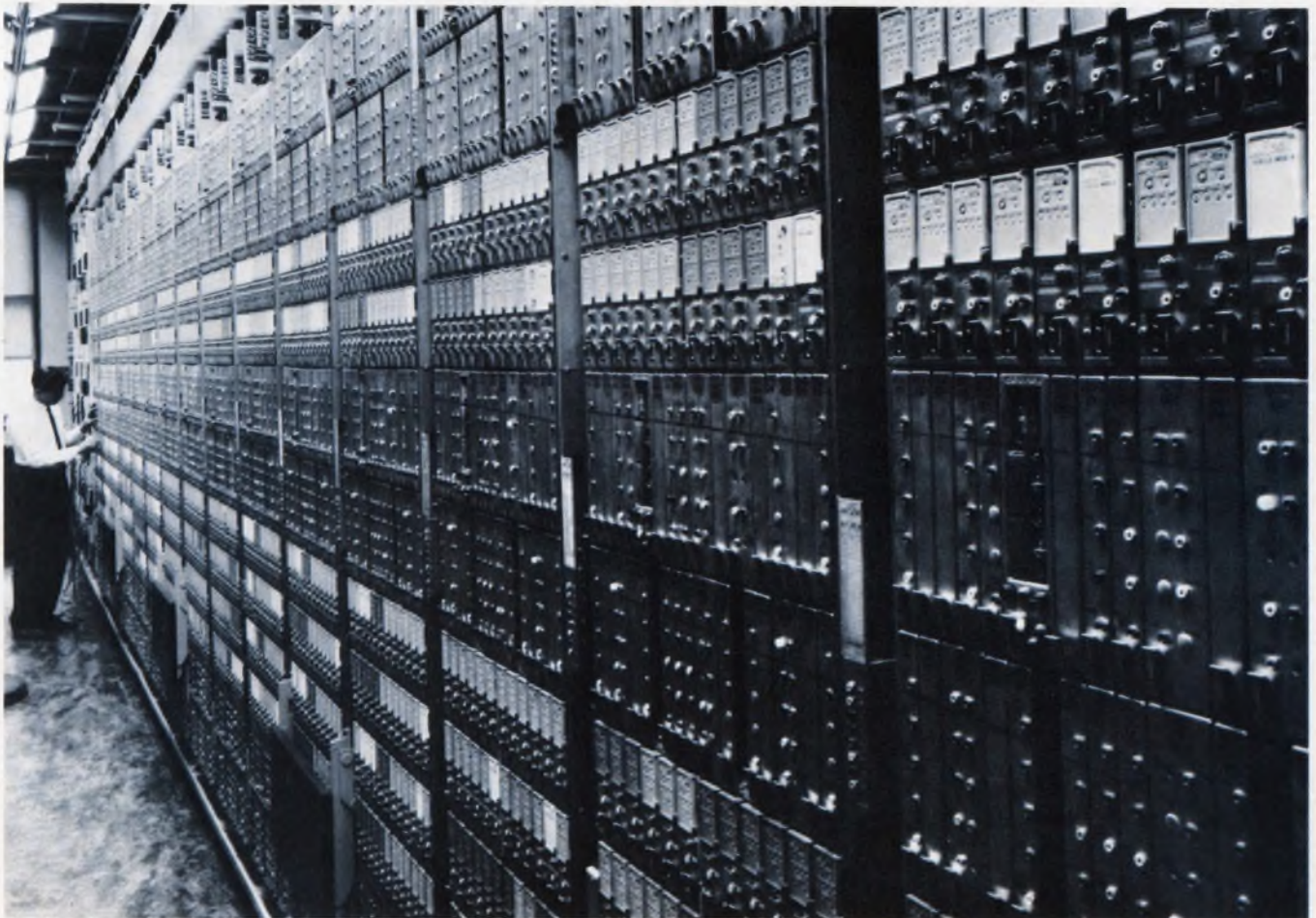
A digital first: These are terminals for Bell's T1 carrier system, which uses PCM to transmit 24 two-way tele-
