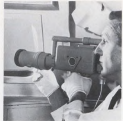
TV camera that sent back views of the moon and earth never seen before weighs 4.5 pounds, uses a 1-inch vidicon tube and pulls 6.7 watts. Built by RCA, it uses a 500-kHz bandwidth and provides 10 frames per second with a 320-line raster.
