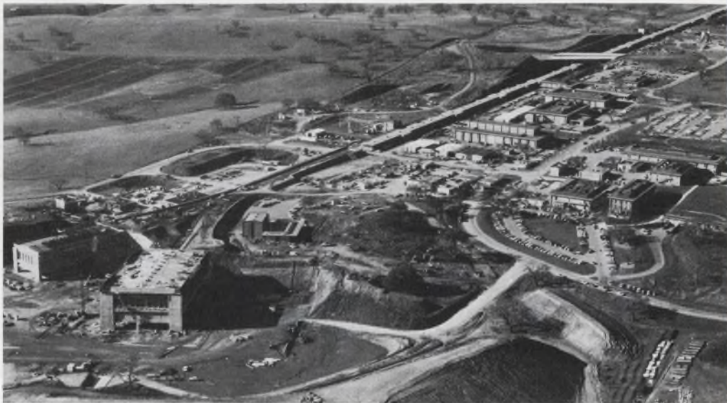
Aerial view of SLAC shows the above-ground portion of the 2-mile-long linear accelerator. The buildings at the left will contain experiments to be bombarded by the 20-GeV (Bev) electrons, which will begin their 2-mile race from the distant end.
