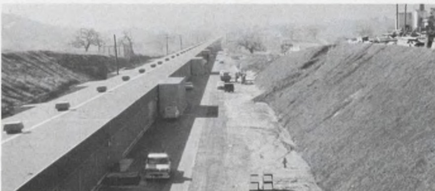
Aerial view of SLAC shows the above-ground portion of the 2-mile-long linear accelerator. The buildings at the left will contain experiments to be bombarded by the 20-GeV (Bev) electrons, which will begin their 2-mile race from the distant end.
