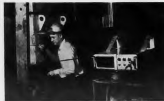
ELECTRO-CHEMICAL ANALYSIS. Savings of as much as $8,000 a year, on one particular project are expected to result from use of an NLS 481 DVM at Diamond Alkali Company's plant in Dear Park, Texas. By accurately measuring small changes in voltage and voltage drop, it permits optimizing the efficiency of producing chlorine from sodium chloride brines by electrolysis.
