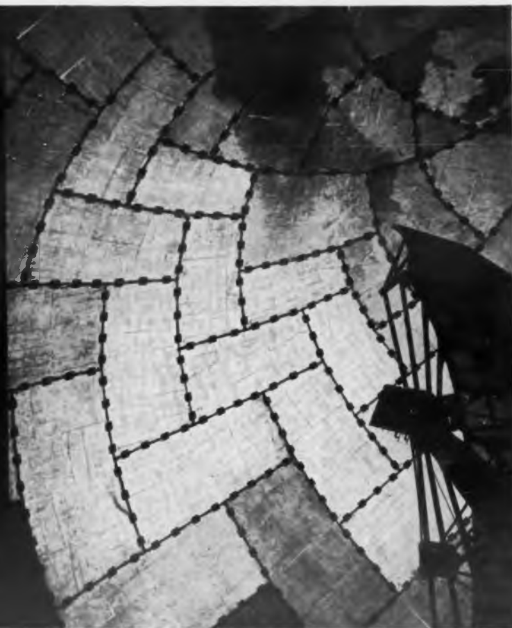
Looking upward from the inside of the world's largest stressed skin sandwich radome built of translucent fiberglass panels, securely joined by hundreds of DUAL-LOCK fasteners.
