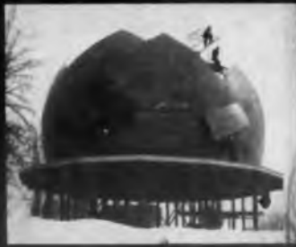
Radome designed and built by Long Sault Woodcraft Limited, St. Andrews East, Quebec, for the United States Air Force RADC.
