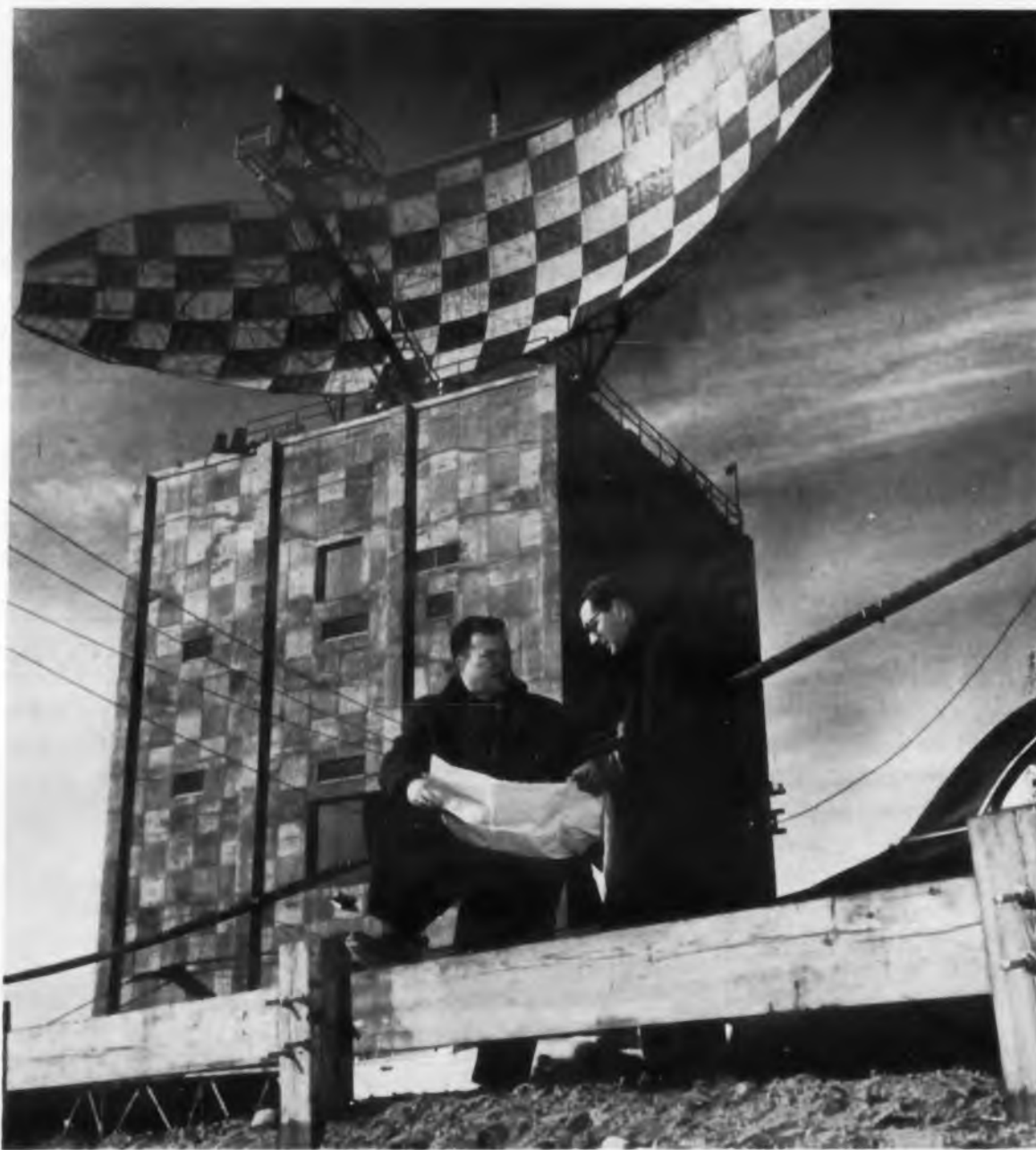
Cold-war psychology demands that the enemy know the U.S. can accomplish projects like the AN/FPS-35 defense radar system within two years. Although the full scope and schedule of this multi-site system are classified, this picture of the second unit at Montauk Point, N.Y., was taken last spring. Sperry engineers Frank Mulligan (left) and Lawson Singer directed the assembly of the Sperry and subcontractor parts sent directly to the site.
