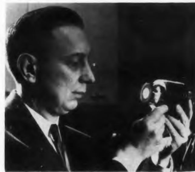
Astracon image amplifier is examined by Westinghouse scientist Dr. J. W. Coltman. Tube employs new thin-film dynodes and may be applied in night warfare devices, astronomy and nuclear science.
