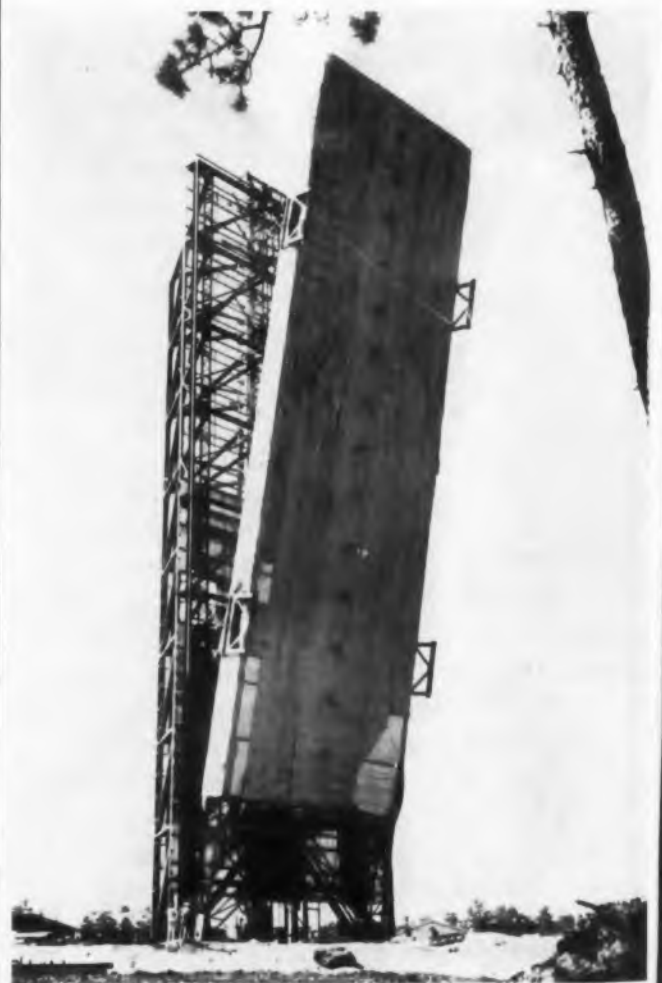
Fig. 6. One of the largest non-military systems, this W. L. Maxson height-finder antenna array, developed for the FAA, when complete, will use 30 miles of waveguide in developing 333 beams.
