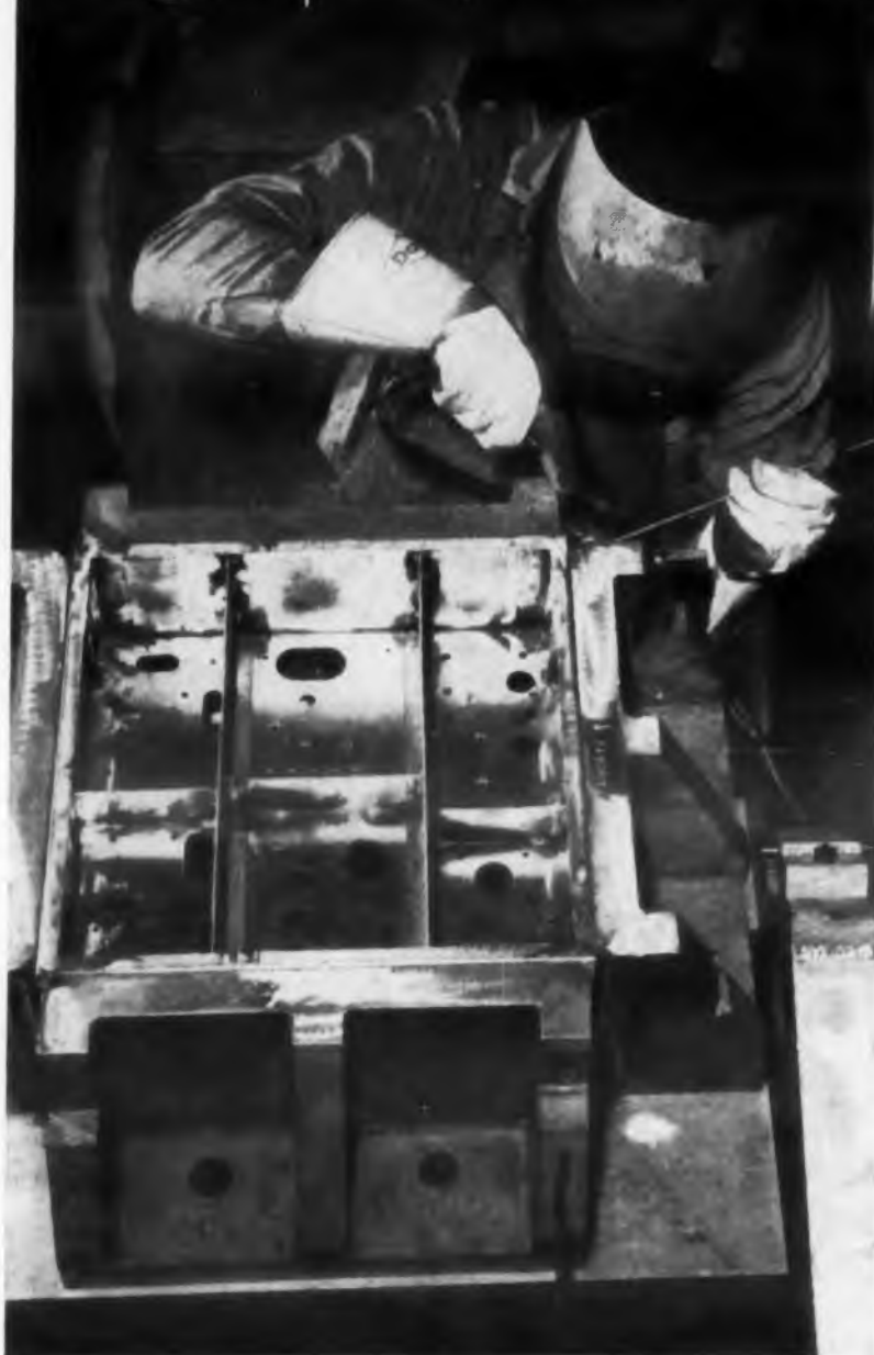
WELDING. Heliarc welding joins parts of this control central case. Dow facilities and personnel for welding are government certified.
