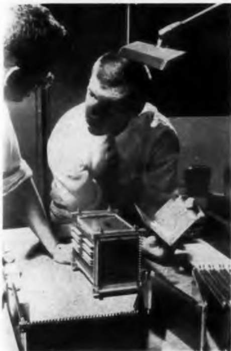
Bell Labsmen H. L. Stadler and D. G. Clemons iron out some fine points of the Twistor memory. A partially assembled module is in the foreground, with a completed unit behind it.
