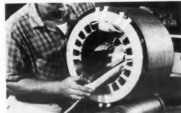
MOTOR SLOT AND COIL INSULATION
