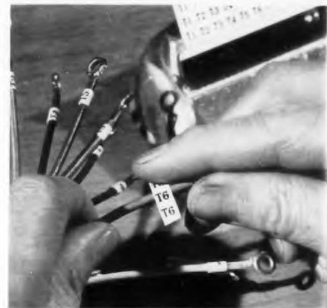
Fig. 15. All leads of this wiring harness are permanently marked with self-sticking markers made by W. H. Brady.
