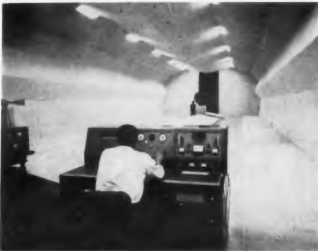
Anechoic chamber is about 120 feet long, 45 feet wide and 25 feet high. The room's frequency range is 900 mc through 50 kmc.
